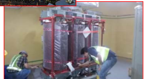
Unpacking the Core & Coils At Site
