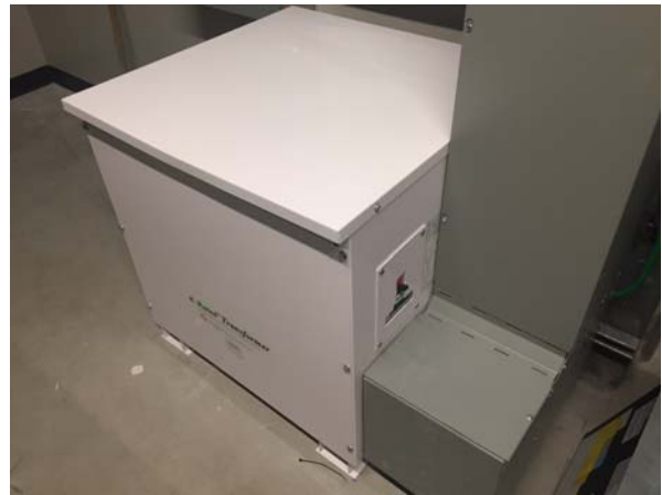
45kVA Power Center™ with Side Mounted Circuit Breakers
